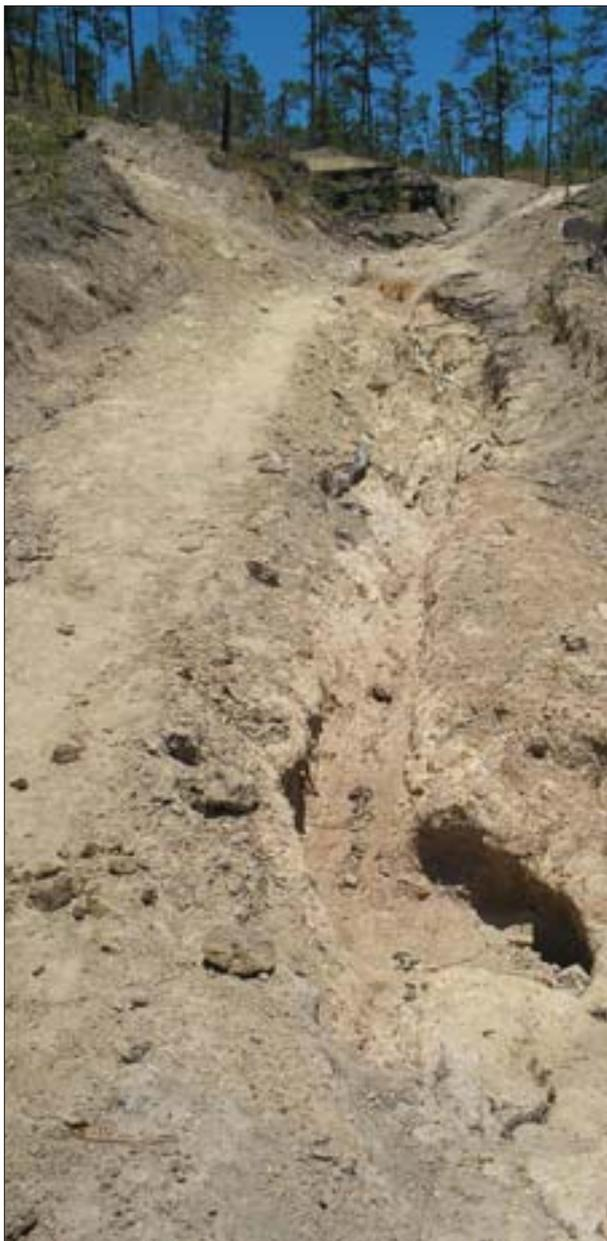
**Pictures 2 and 3. Ruts caused by run-off water on tracks**
